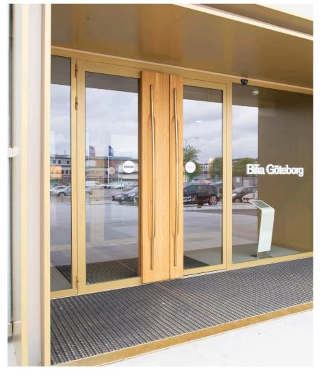
Bilia in Sisjön, Gothenburg, is the world's largest all-Volvo facility and the first global pilot facility for Volvo Car Groups. For the entrance, we supplied steel profiles from systems SP 56500 and SP 35000, which were powder coated in a selected color.
